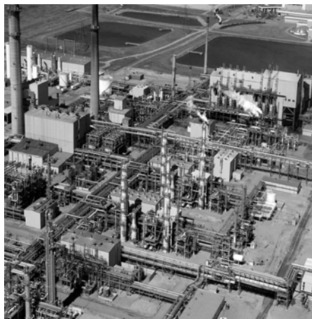
Fig. 4. A pre-combustion CO 2 capture system used to produce synthetic natural gas (syngas) from coal at the Dakota Gasification Plant in North Dakota. About 3 Mt/y captured CO 2 is currently transported by pipeline to the Weyburn and Midale oil fields in Saskatchewan, Canada, where it is used for enhanced oil recovery and sequestered in depleted oil reservoirs. (Photo courtesy of US Department of Energy)
